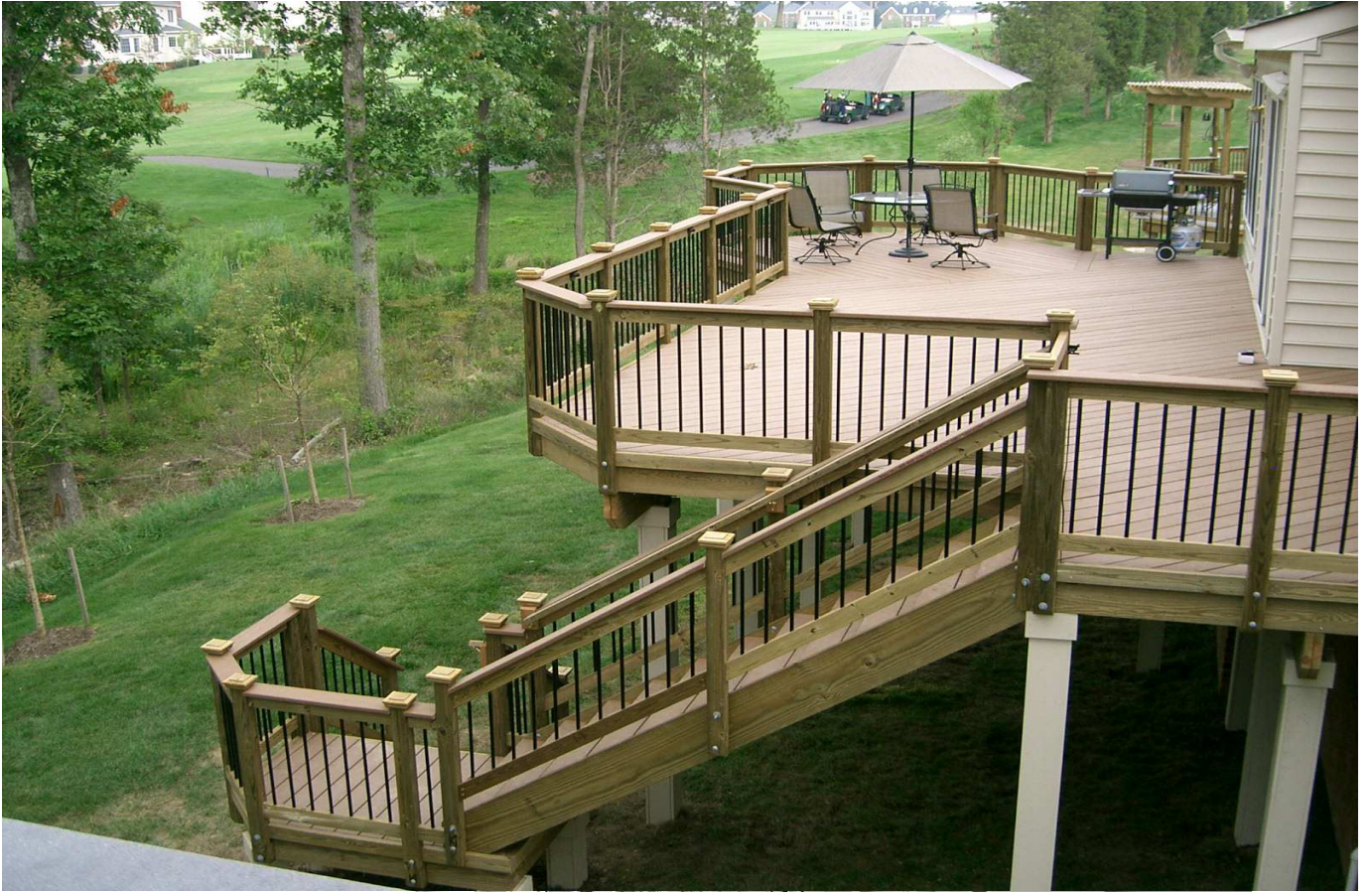
BLACK SPINDELS, WITH POST CAPS, TREX FLOOR, 6X6 POSTS
