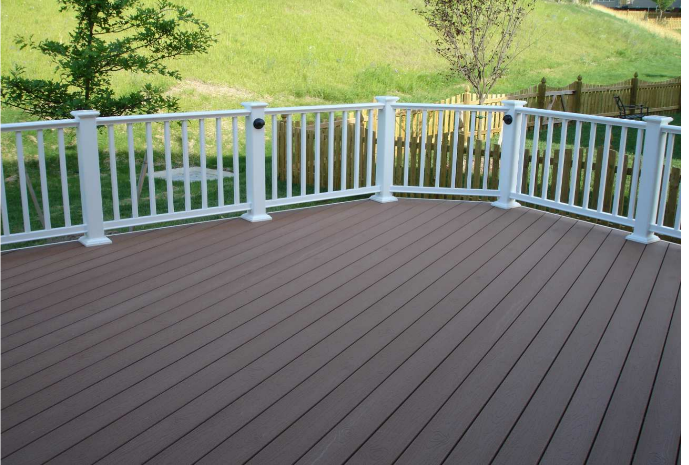
HIDDEN FASTNERS ON DECK FLOOR/ WHITE VINYL RAILS/ LIGHTS ON RAILS
