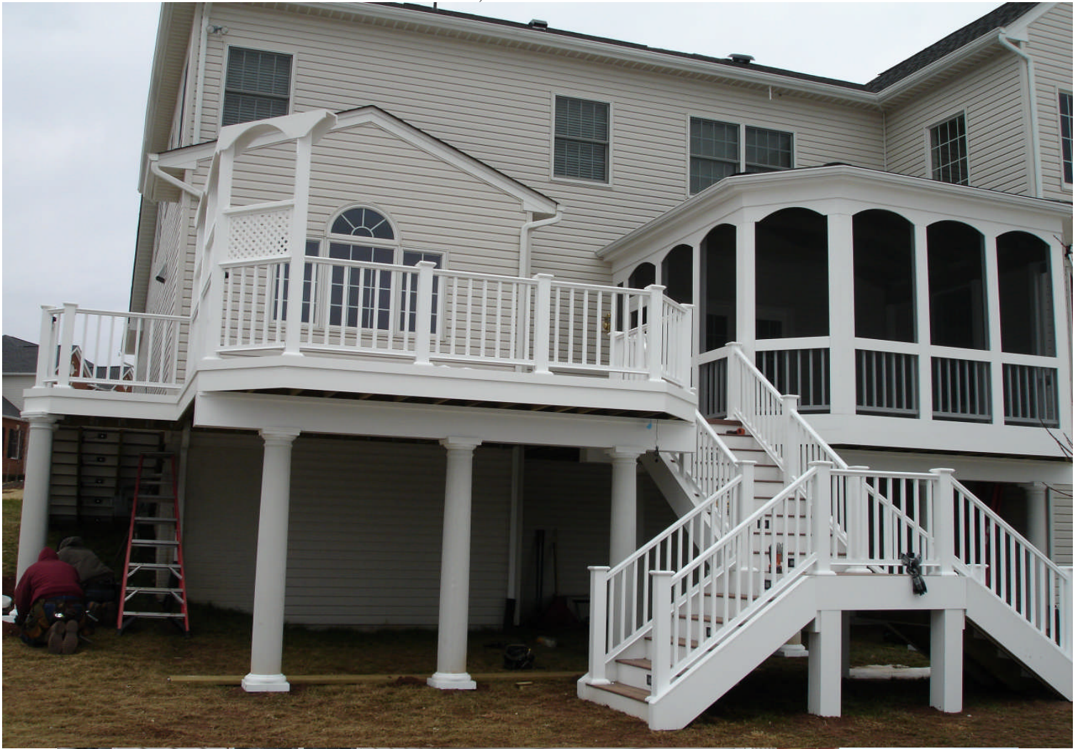
ALL WHITE COMPOSITE DECK AND PORCH, SUPPORT BEAMS UNDER DECK WRAPPED WITH VINYL
