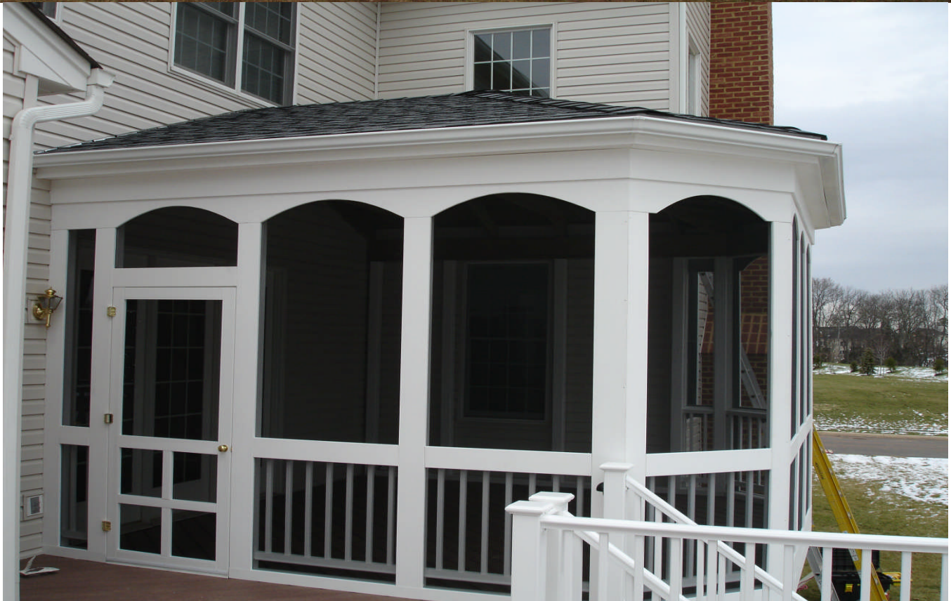
WHITE VINYL TRIM ON OUTSIDE OF PORCH, WHITE COMPOSITE RAILINGS
