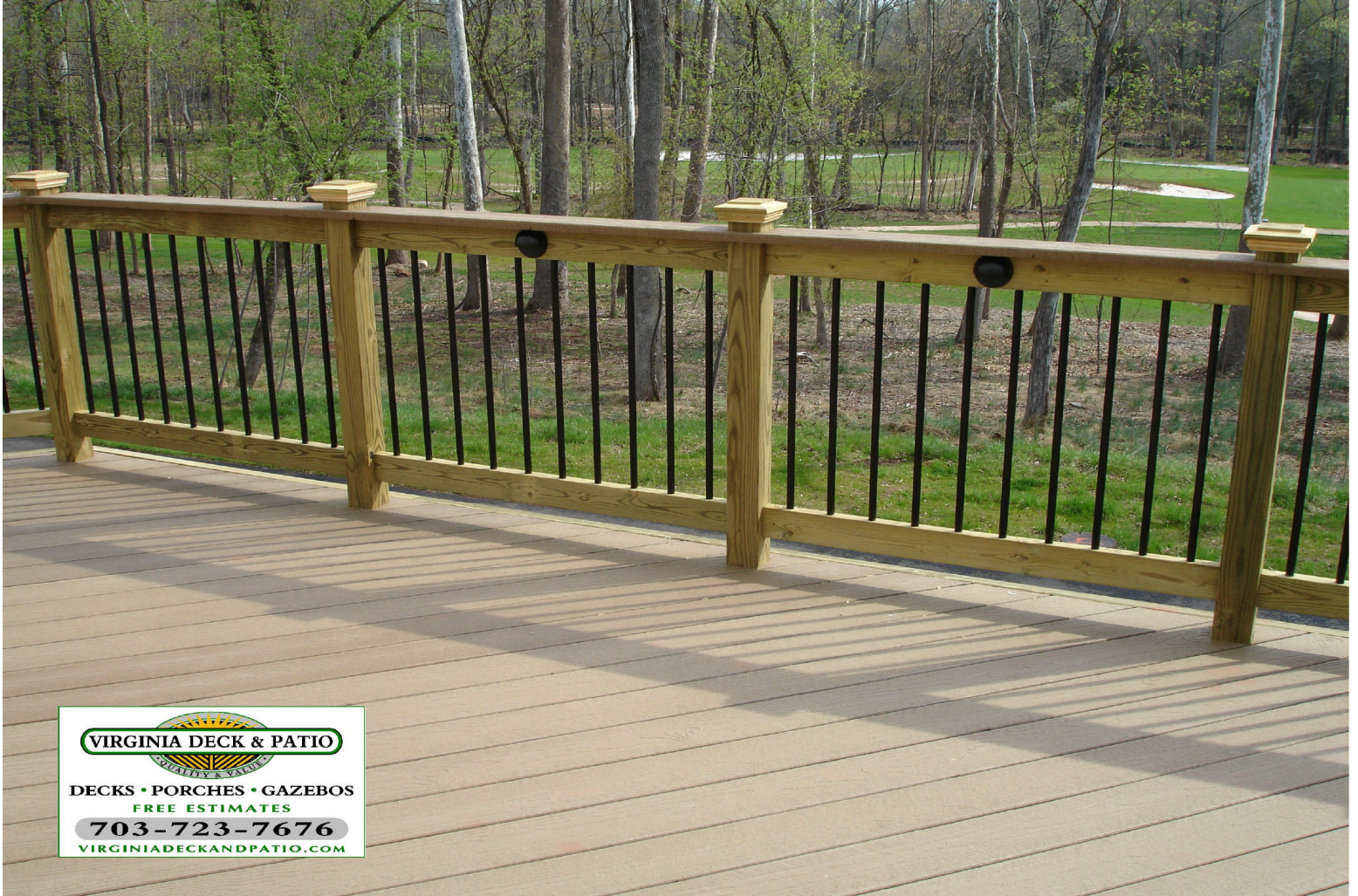
WOOD RAILS WITH BLACK SPINDELS, POSTS ARE INSET, HIDDEN FASTNER, LIGHTS IN RAILS
