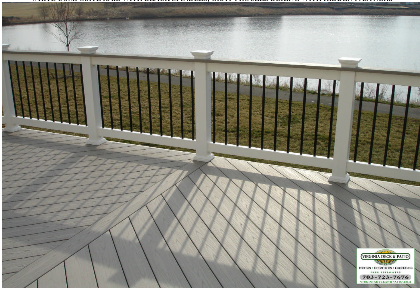
WHITE COMPOSITE RAIL WITH BLACK SPINDELS, GRAY PROCELL DEKING WITH HIDDEN FASTENERS
