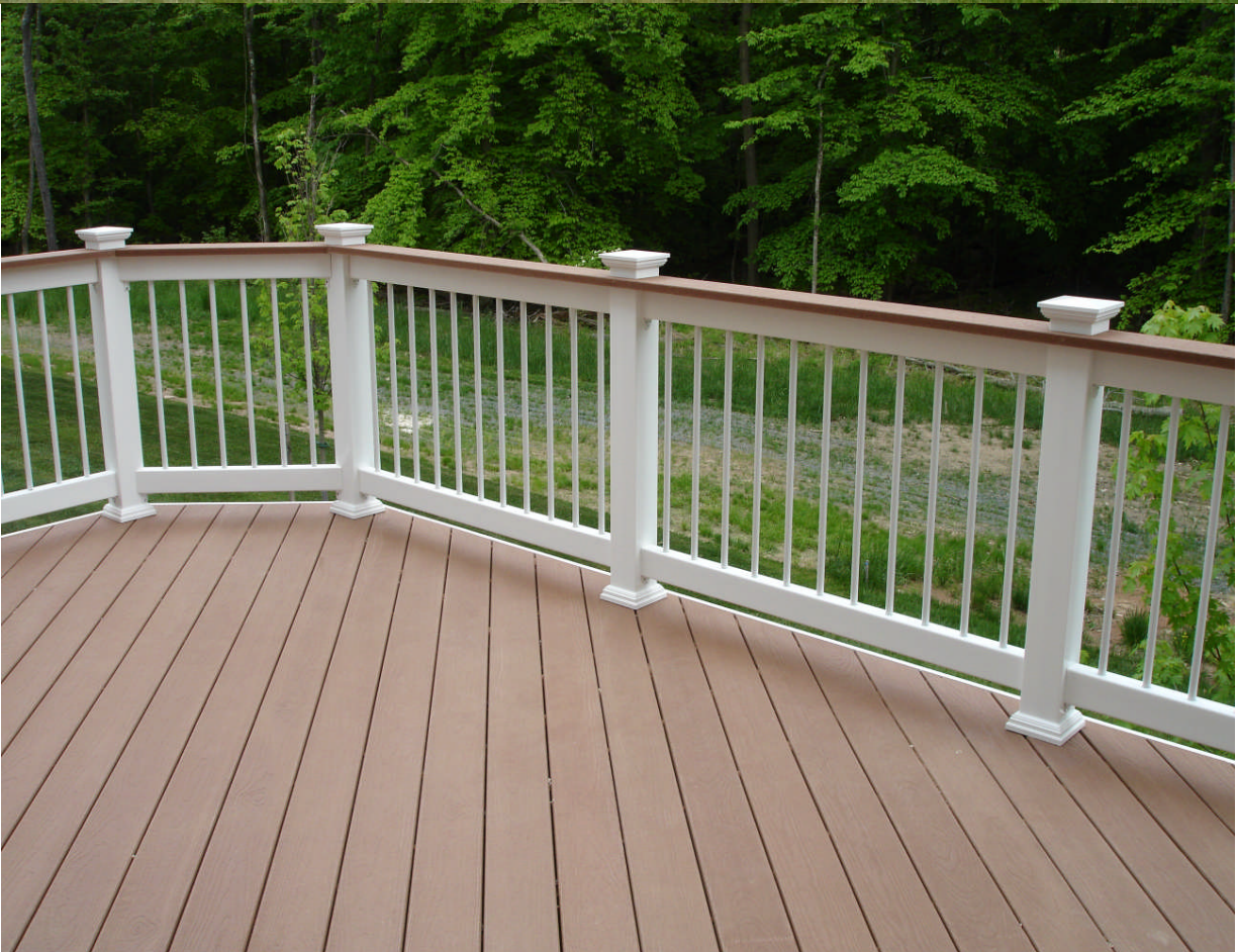
REDWOOD EVERGRAIN WITH HIDDEN FASTNERS, ALSO WHITE COMPOSITE RAILINGS WITH DECKING ON TOP HANDRAIL
