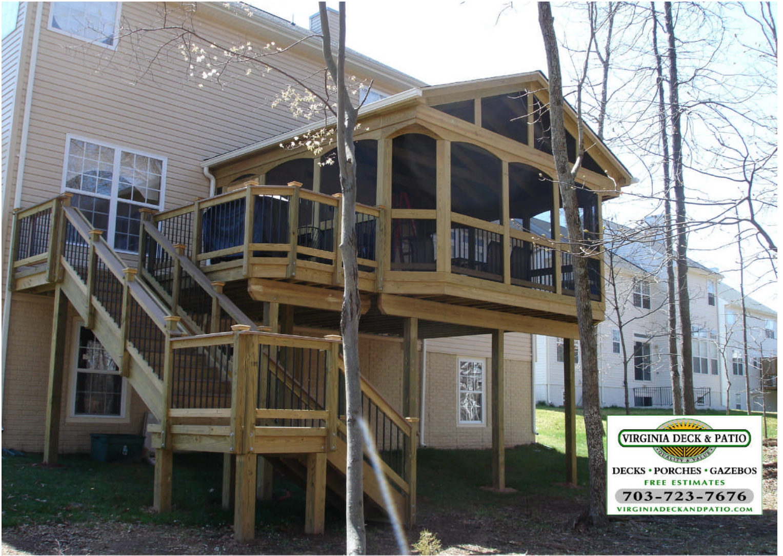
GABLE END WOOD SCREEN PORCH WITH BLACK SPINDELS ON RAILINGS
