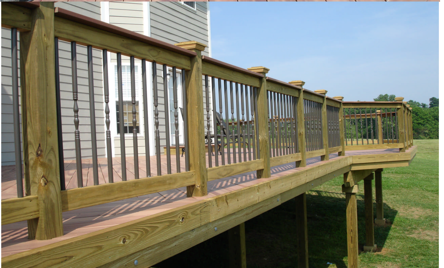
INSET RAILING POSTS/BRONZE COLONIAL SPINDELS
