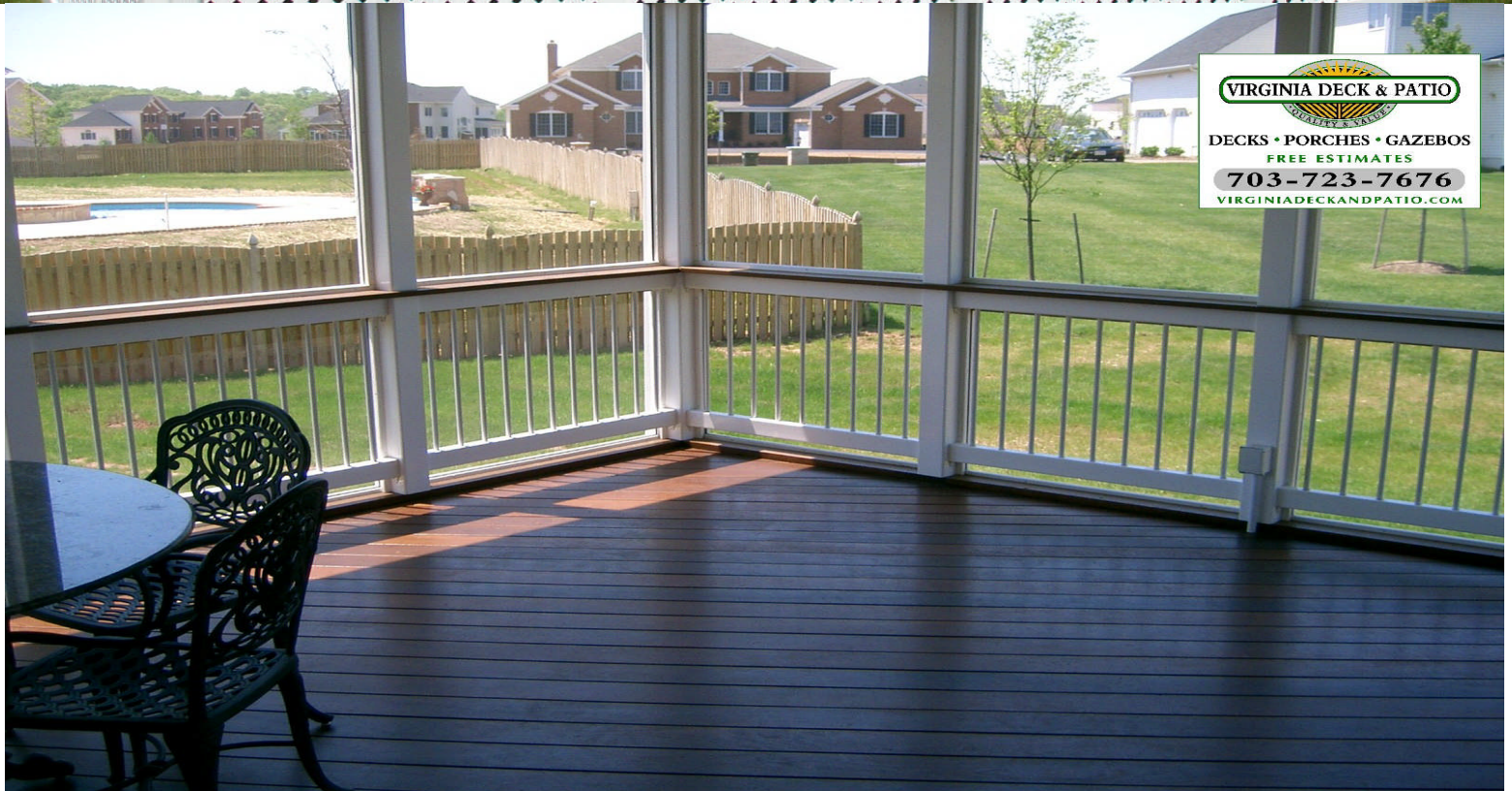
INSIDE PORCH WITH "IPE" WOOD FLOOR AND WHITE COMPOSITE RAILINGS
