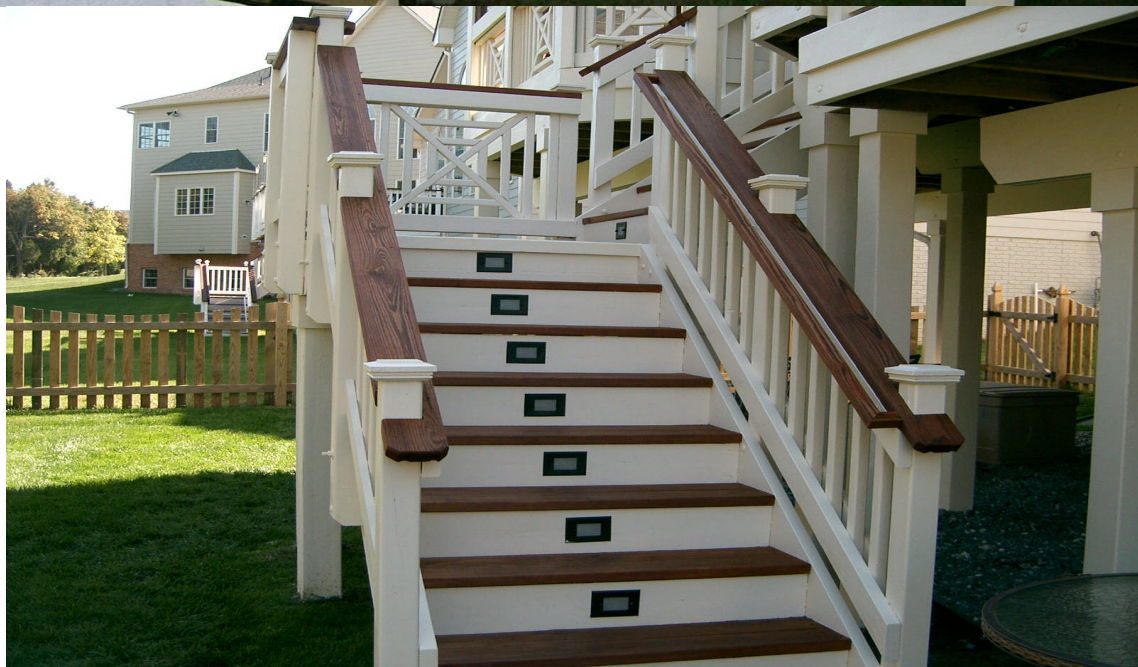
LIGHTS IN STAIRS
