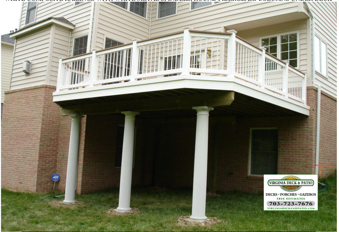
WHITE COMPOSITE RAILINGS WITH WHITE METAL SPINDELS, ROUND FIBERGLASS COLUMNS UNDER DECK
