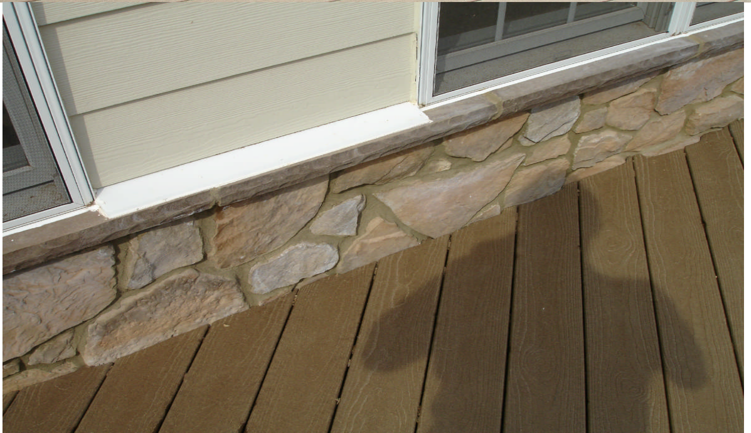
TIGHT CONTOUR CUTS OF FLOORING , AROUND STONE WALL, HIDDEN FASTNERS
