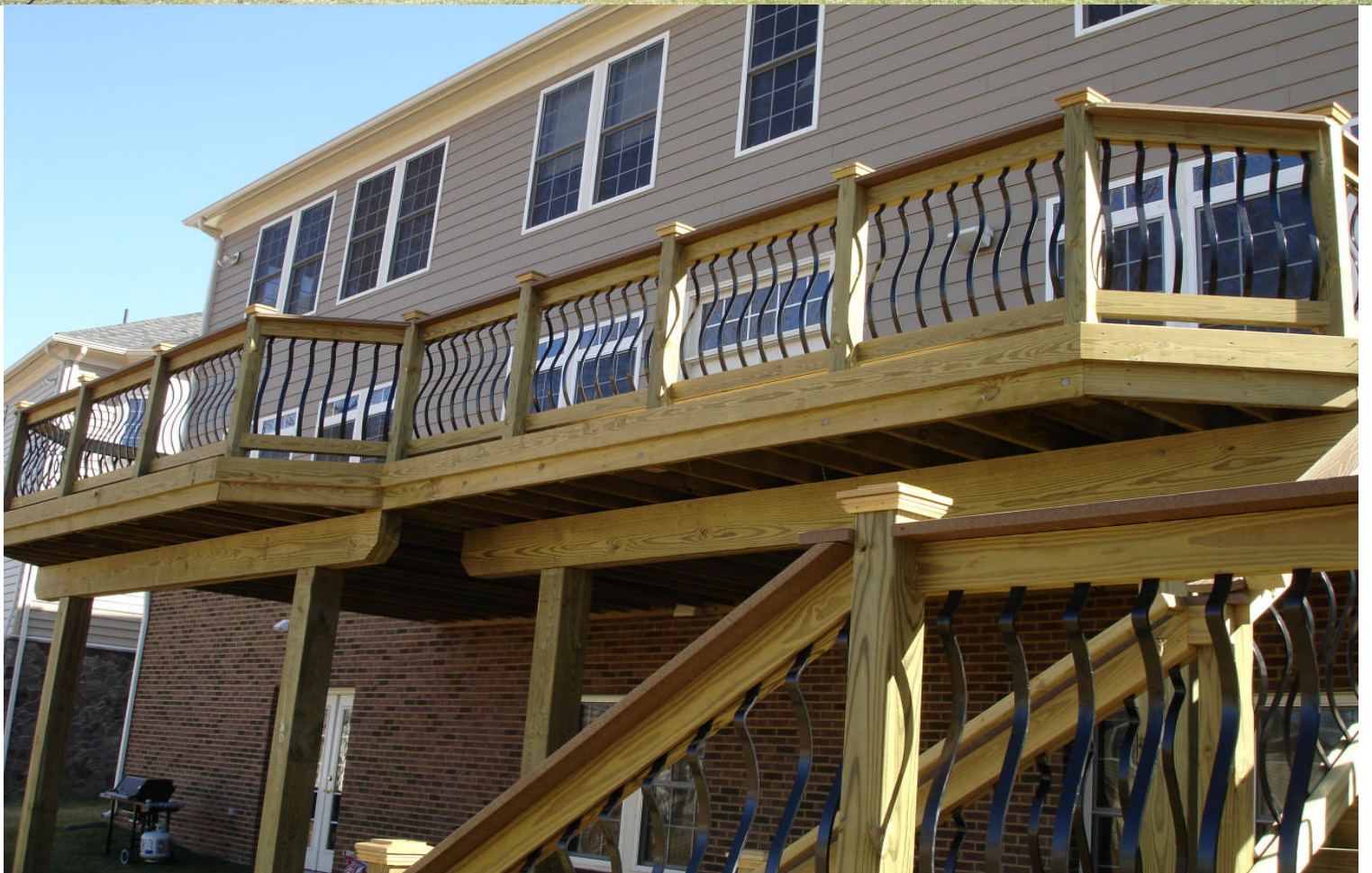
RAILING POSTS ARE INSET,, ON TOP OF DECK FOR CLEANER LOOK, BAROQUE STYLE BALLUSTORS
