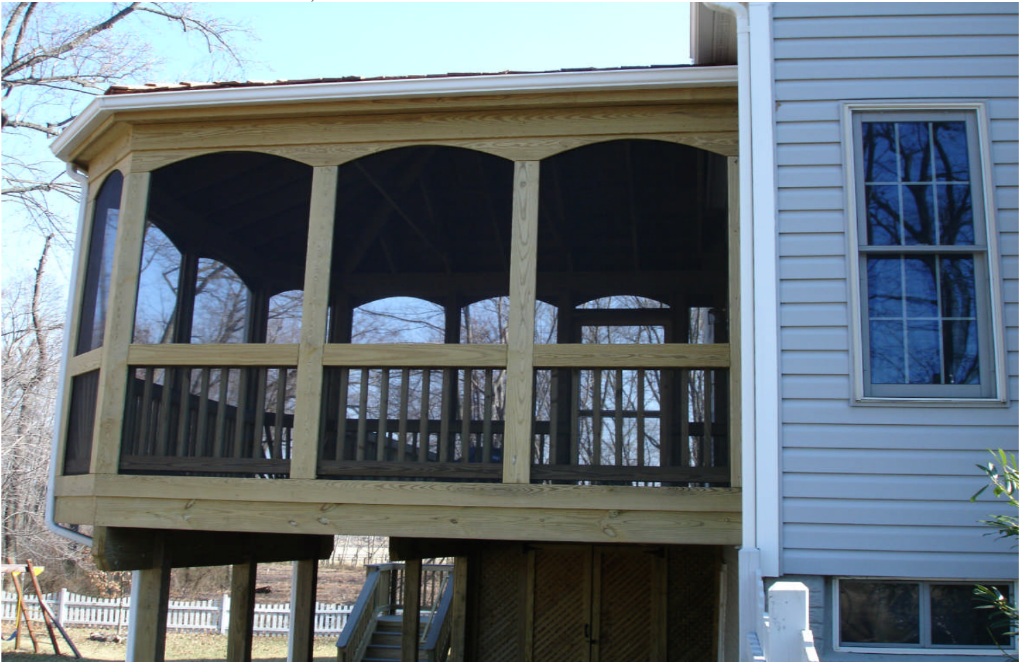
HIP ROOF , WOOD RAILS AND WOOD TRIM ON OUTSIDE OF PORCH
